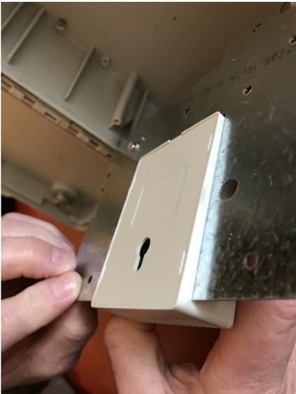
4. Use a flat blade screwdriver to open receiver box.
