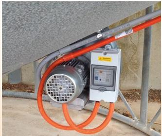
Start boxes have a contactor to start and stop fans with overload, Earth leakage and lightning proof protection and are capable of running 4-6 fans on a 10 amp lead. This allows one controller to aerate dozens of silos.
