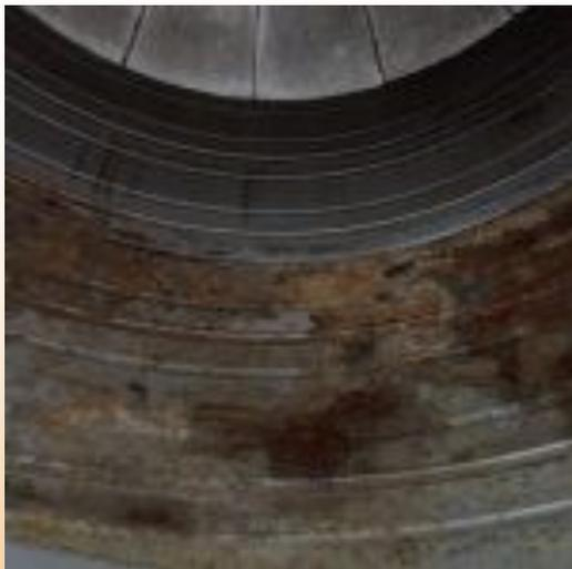
Note the corrosion to the walls in this near new 109t silo caused by damp grain. This silo was filled with grain at harvest that had too much moisture that condensed to the silo roof then ran down the silo walls.
